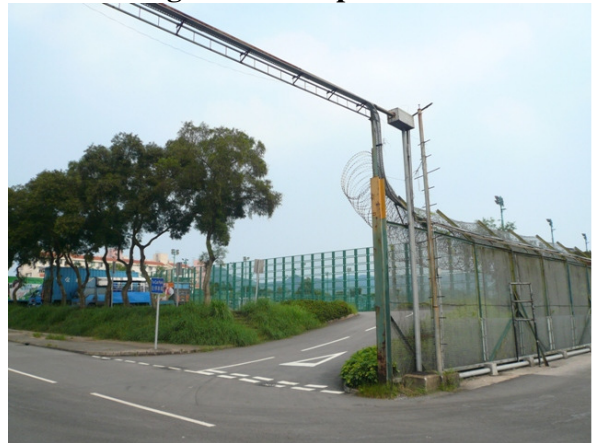
Plate 12 Proposed site for the new GATE ONE Checkpoint
