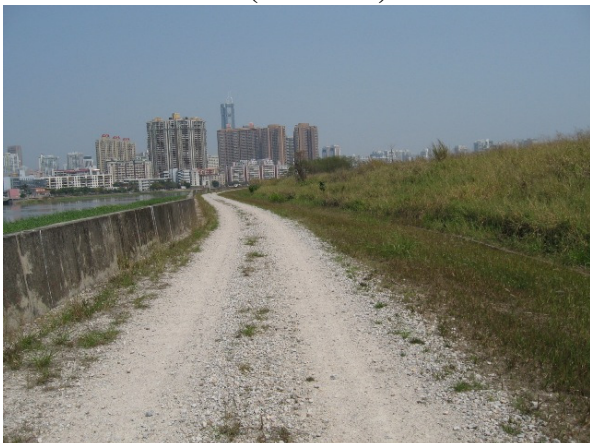
Plate 5 Drainage Maintenance Road located at the north of Lok Ma Chau Loop (Section 2)
