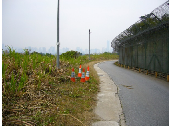
Plate 2 Boundary Fence to be removed in Lok Ma Chau (Section 2)
